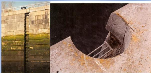
Recessed quay wall ladder with coping stone that was extremely difficult to climb over at the top and (right) semi circle cut into stone to allow easy climbing.
